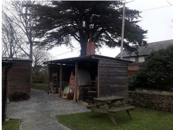
Figure 2. Open fronted store/kiln
