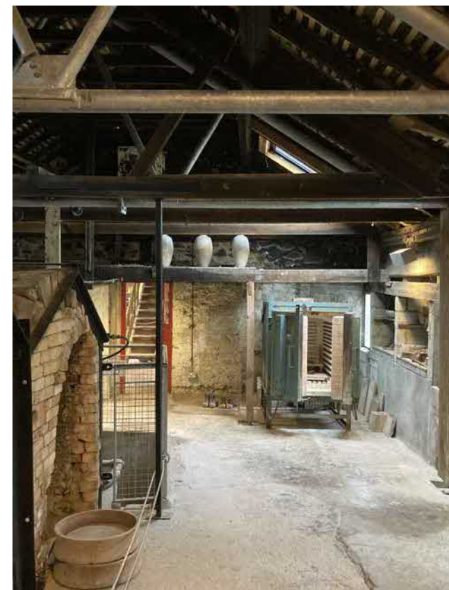
The kiln room
