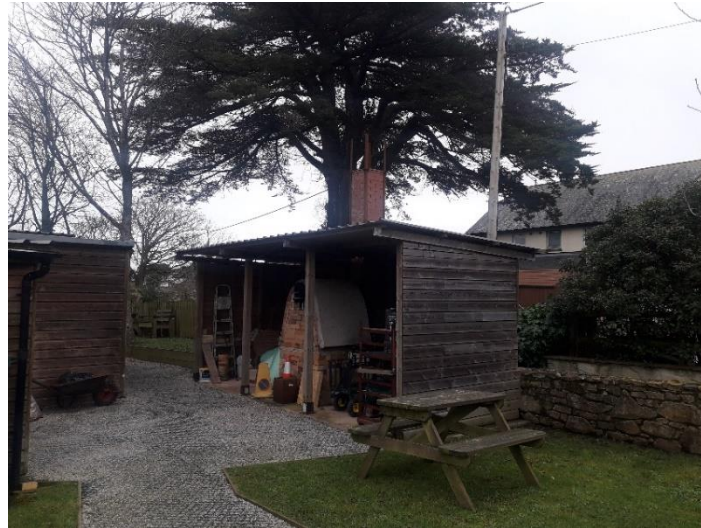
Figure 2. Open fronted store/kiln
