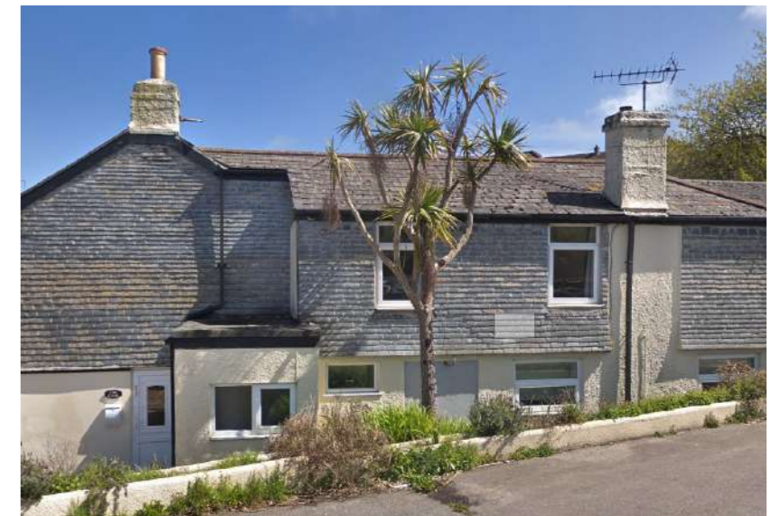
Far left: Garden Museum London, a contemporary version of copper shingle cladding Top left and right: Porthmeor Road, St Ives, a granite plinth with slate walls and roof Above right: Penbeagle Lane, St Ives, (next door to the pottery) slate walls and roof Left: slate grey zinc shingles
