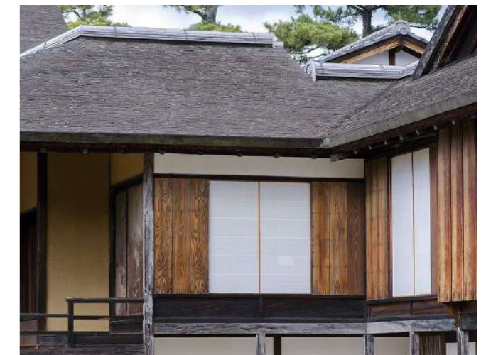
Top: Plan of the Katsura Palace Above: The pitched roof forms of the Katsura Palace Left: Deep threshold spaces to nature
